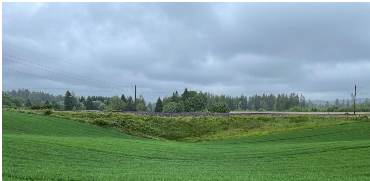
Figur 9: Jernbanefylling i ravine.
